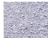
Rough Plaster Wall
